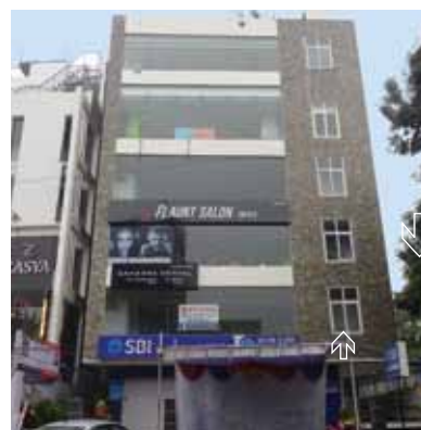
Dr. YV Rao Hospital (Hospital Lift installed)
